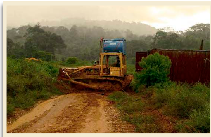
ACCESS ROAD PREPARATION - MONTAGNE D'OR
