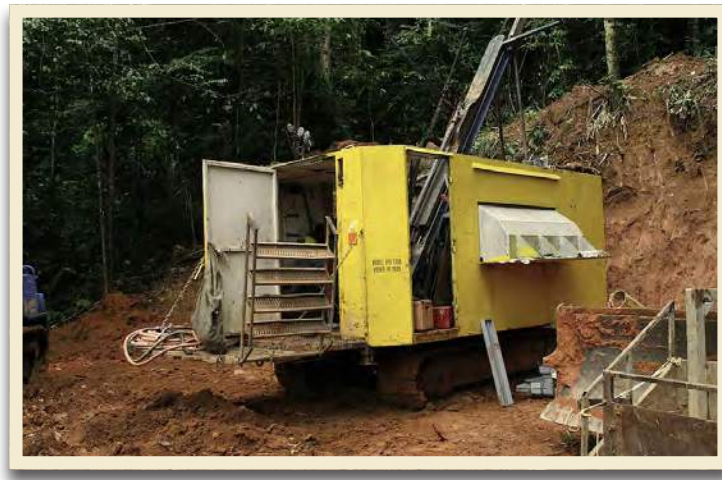
TYPICAL HILLSIDE DRILL SETUP - MONTAGNE D'OR
