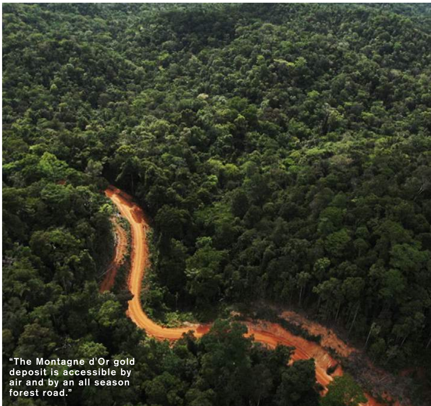
Photo: Forest road from the port city of Saint Laurent du Maroni to the Montagne d'Or gold deposit - Paul Isnard gold Project, French Guiana.
